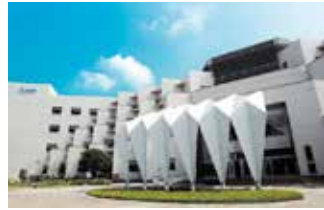
Tainan Plant (Diamond-rated Green Building)
