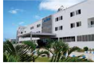
Rudrapur Plant (Green Building)
